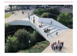
opposite trapeziums. The trough-based structural principle provides visual and acoustic protection to the walking area of the footbridge. It also makes it possible to give it two solid railings, whose height just about allows a horizontal view.
